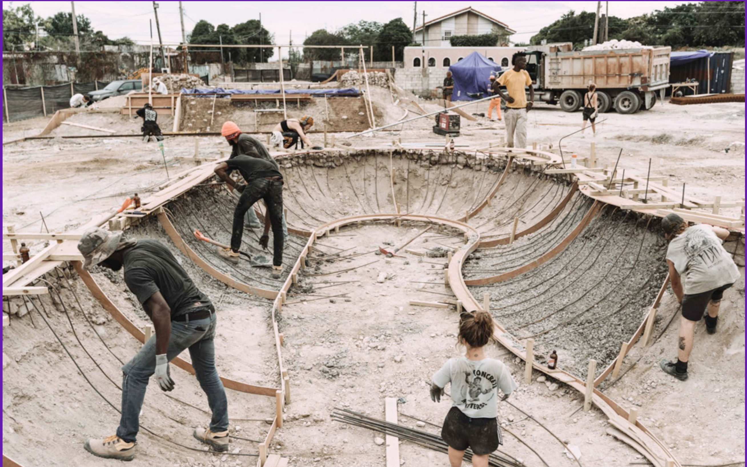
The Freedom Skatepark in Jamaica being built in spring 2020. Credit: Ayden Stoefen for the Concrete Jungle Foundation
